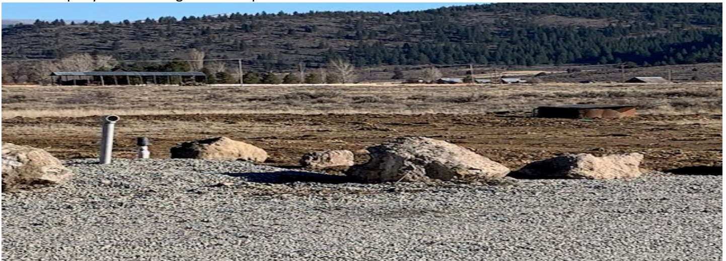
Stand pipe access to the underground water tanks and the helicopter dunk tank in distance
